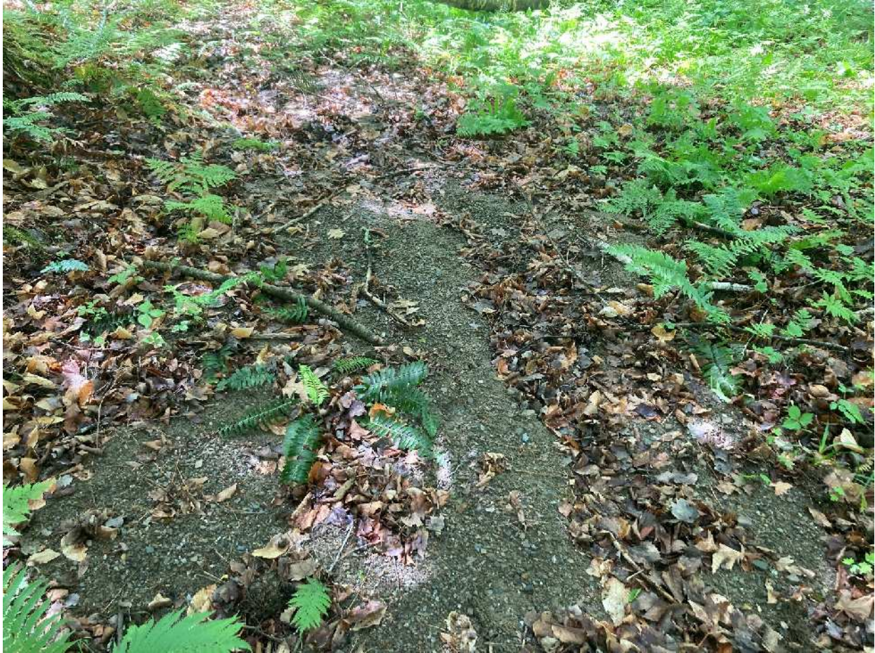
Figure 2. Sediment from the trail surface deposited downhill by the stream channel. Some of this sediment made its way directly into the stream channel. In this area, a second channel is eroding parallel to the stream channel. Further erosion could result in the stream “capturing” the old logging trail.
